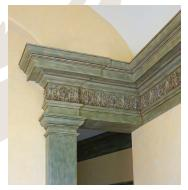
14" wide Tuscan column is sheet-rocked and has the identical finish as entablature that it supports.
